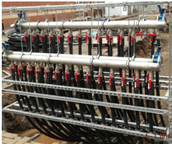
Figure 14. GLHE Manifold
