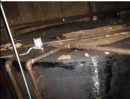
Figure 2. Wax tank for thermal storage
